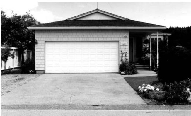
There is little in this design to draw the eye away from the garage door. The design lacks a residential emphasis.
