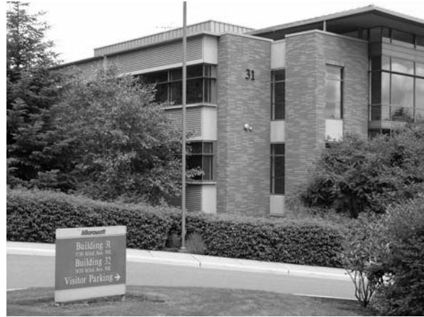
Microsoft building – LEED certified
